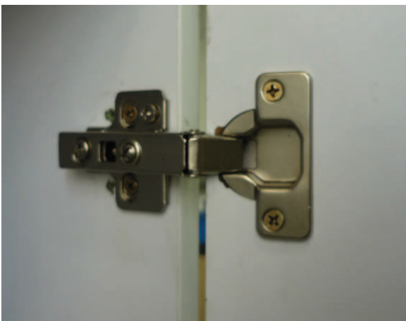
Pic. 3: Hinge mounted on a cabinet (2)
