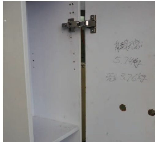
Pic. 2: Hinge mounted with a door (1)
